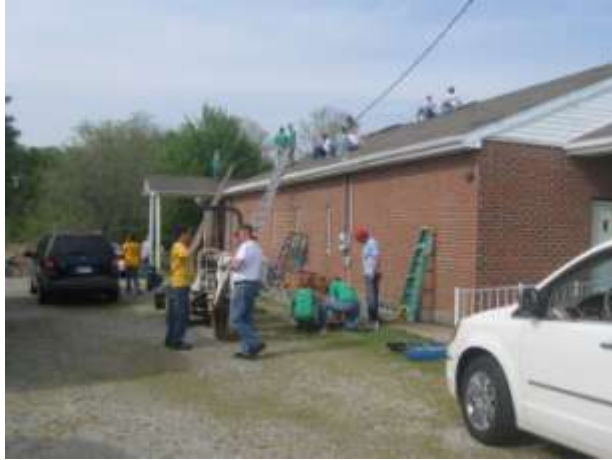
Preparing the lift and gathering shingles to move to the roof.
