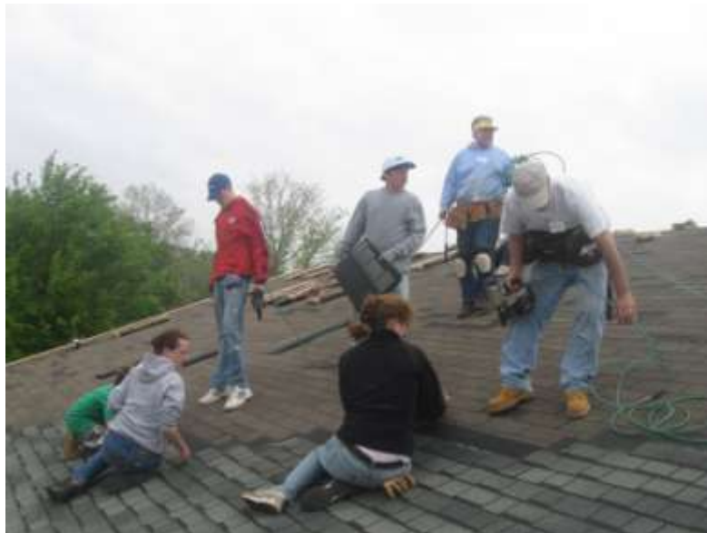
Newly-trained roofers installing the new shingles
